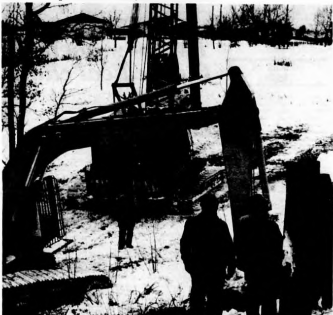
Nelson River Construction drive 30 ft. piles into the side of Highway #11 near #304 prior to installing an 8 ft. square culvert to correct the sagging road.
