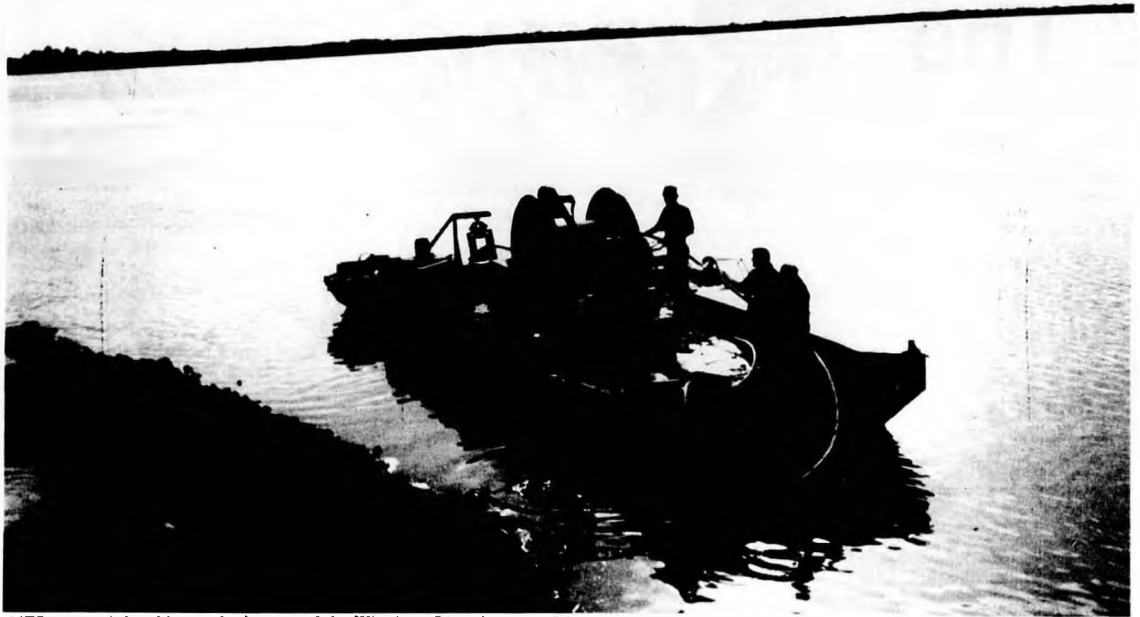
MTS crews sink cables to the bottom of the Winnipeg River between Silver Falls and Broadlands Road to install private lines for grateful customers.
