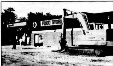
Preparing the base for paving.
