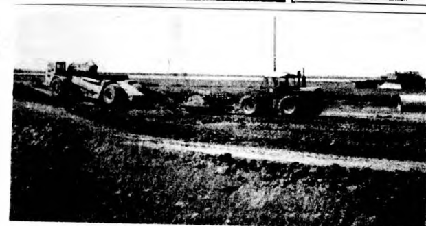
Construction is underway on the re-direction of Highway 304. The new route will by-pass Stead.
