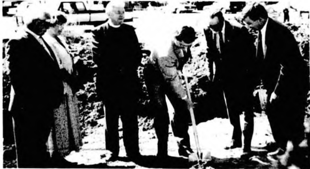
Provincial Health Minister Don Orchard turns the first sod to officially launch the construction of the $1.63 M personal care home. Looking on is M.L.A. Darren Praznik (right) and others.
