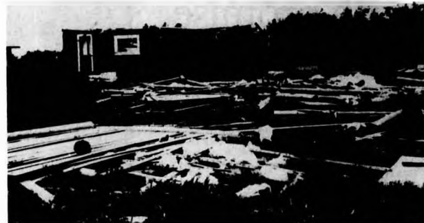
One example of the destruction caused by the June 24 storm. This cabin at Leisure Falls lost its roof while some others were completely destroyed by the high winds which reached speeds of up to 150 km/h.
