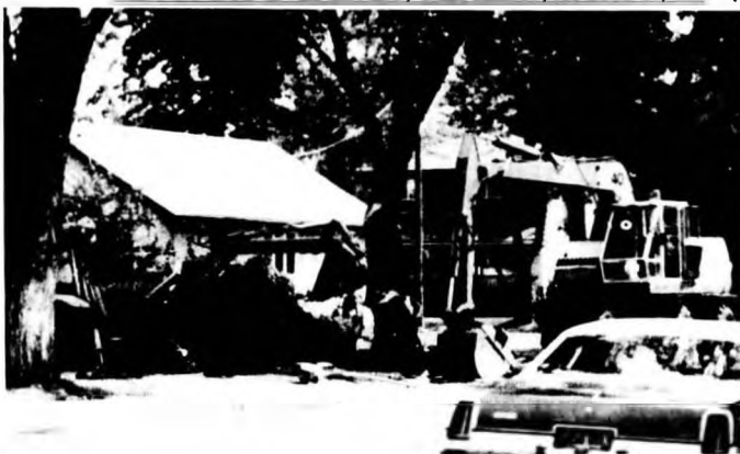
A crew work to replace a hydrant while sewer and waterlines are being changed. This construction caused water to be off for two days last week in Pine Falls.
