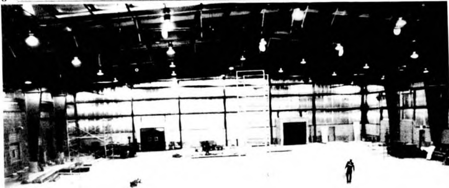
The new Abitibi paper warehouse is quite the size. Overall floor dimensions of 225 feet by 133 feet and the roof reaches 32 feet to the peak. The warehouse hopes to be storing finished paper products within a week or two.
