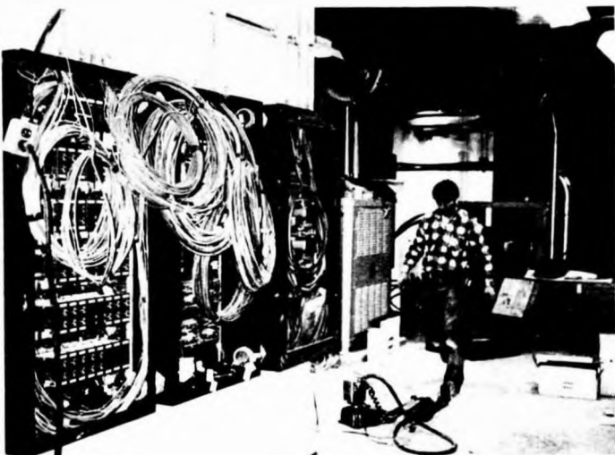
Electrician putting the finishing touches to some of the intricate network of electrical panels. These three are for the alarm system alone for the complex.
