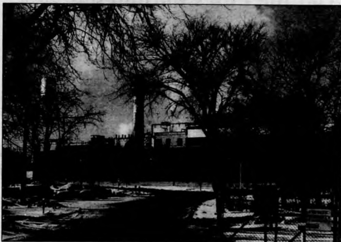
The Tembec Mill in Pine Falls
