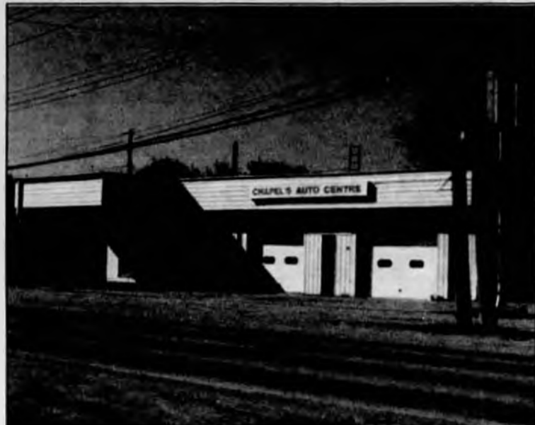
According to Council, Don Chapel's building (pictured above) will not suit their future needs.
