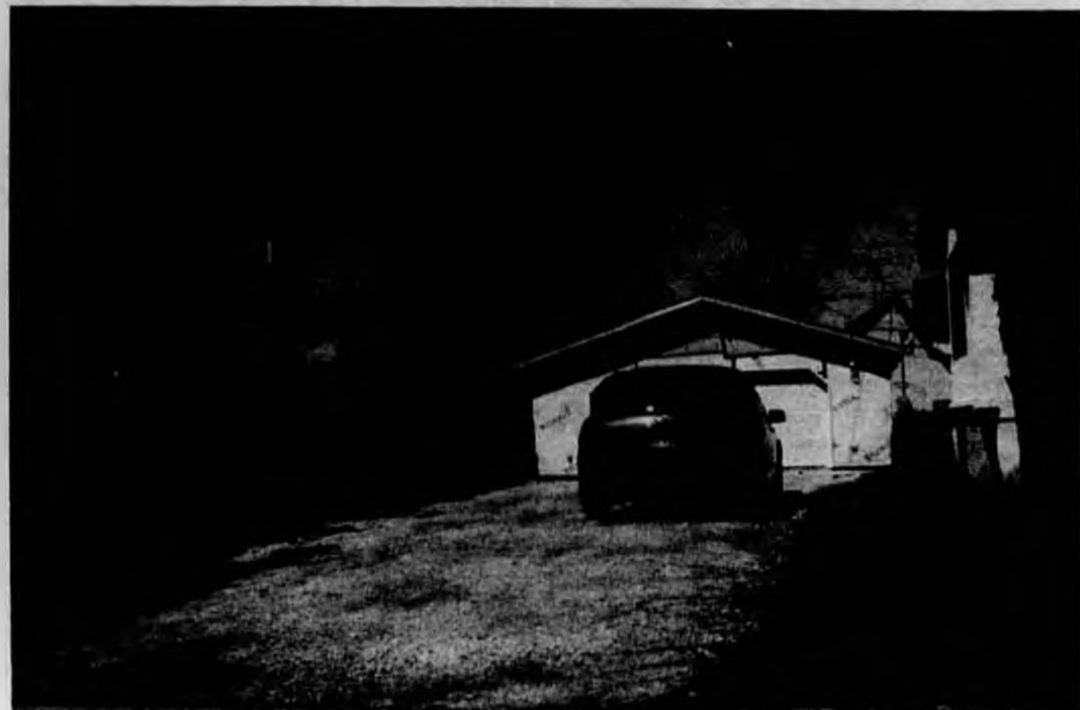
Sean Kemball's Garage. The public right-of-way still runs right through it, in spite of the footpath being moved
