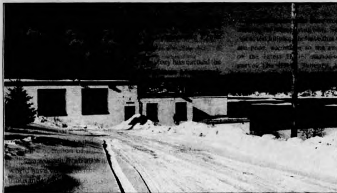
Water treatment plant in Pine Falls
