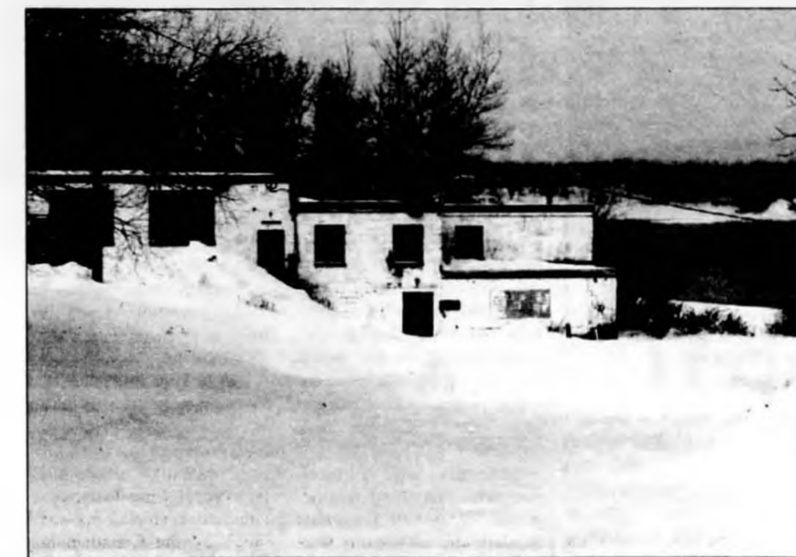
Water Treatment Plant in Pine Falls
