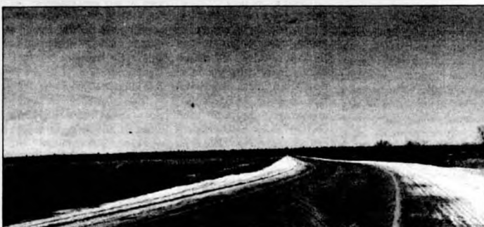
This section of Highway 59, alongside the hillside lagoon will probably be the last to be twinned, perhaps in 2017
