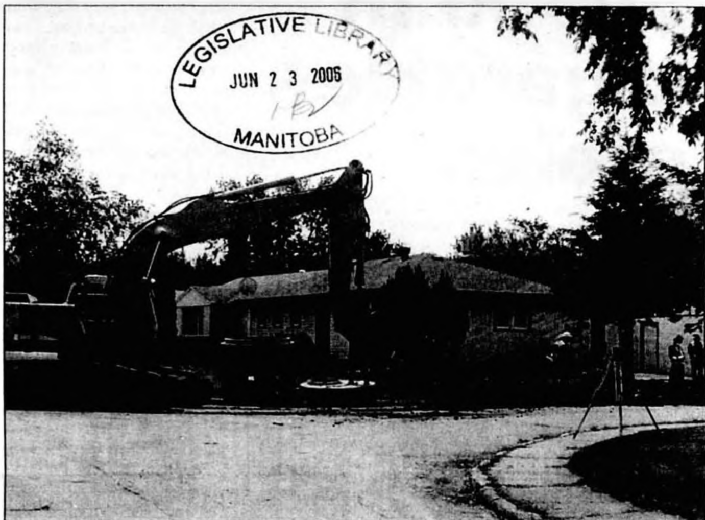
Work on the storm sewer system in Pine Falls is expected to be completed in six weeks.
