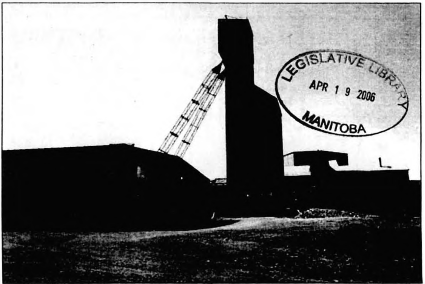
The new head frame at Bissett's Rice Lake Mine
