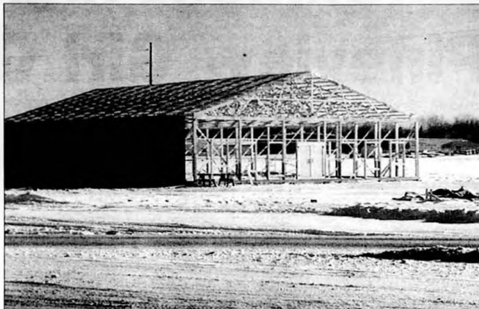
The new Powerview Auto Supply building under construction on Highway 11 & 304
