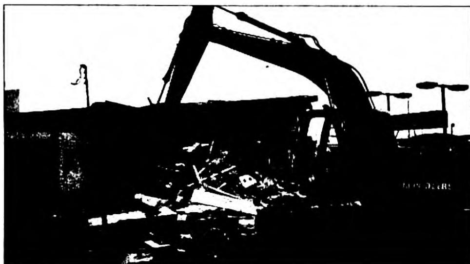
Arsenaull Trucking made the old Tangle Ridge building disappear in rapid fashion last week as the CO-OP convenience store moved into its new location just a few feet away.
