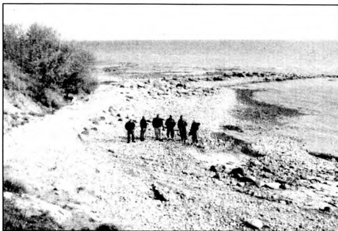
Three erosion protection projects, are in the design stages. One in Traverse Bay, Winnipeg Beach and Hnaua
