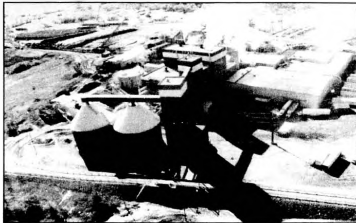
Tembec TMP Plant (file photo)
