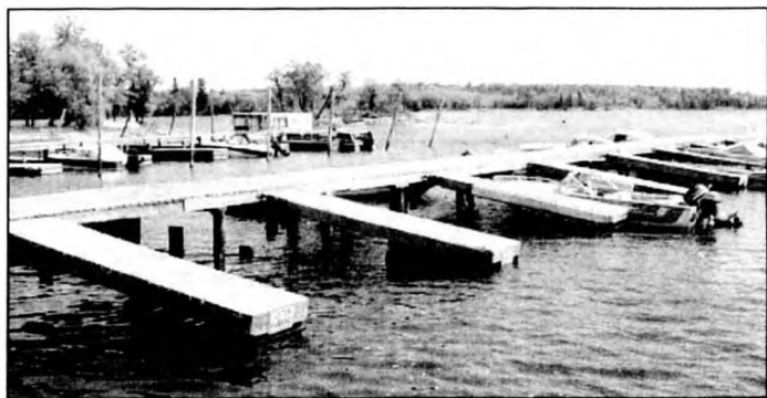
These floating docks in the Whiteshell Park normally sit horizontally with the main pier but low water levels have turned the side mounted structures into ramps
