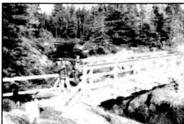
The Blue Water bridge that was constructed this past year
