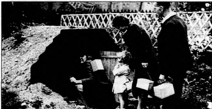
A typical World War II Anderson Air Raid Shelter
