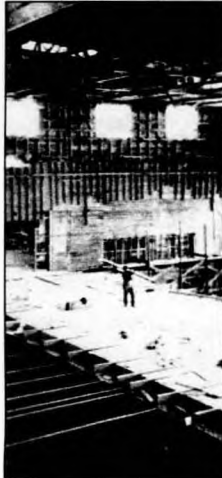
The Mill under construction 1926
