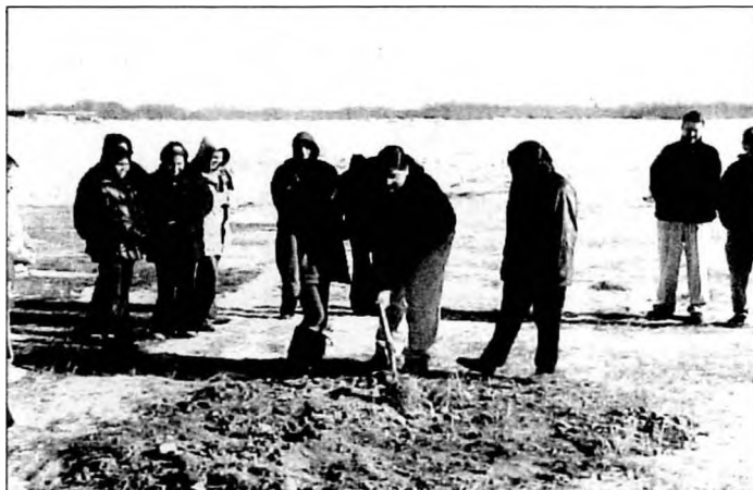
Chief Gary Swampy (centre) marks the official site for the new Sagkeeng Elementary School. The school is planned to begin construction within the next couple of weeks on the old powwow grounds at the east side of the community.
