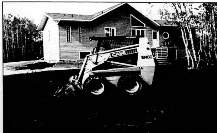
Art Johnson, of The Concrete Works, spreads and levels top soil at Calvin, Sheri and Dane Hirst's residence on Whitecrest Road.
