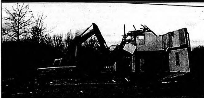
The Bouvier store in St. Georges being demolished on Friday, November 6
