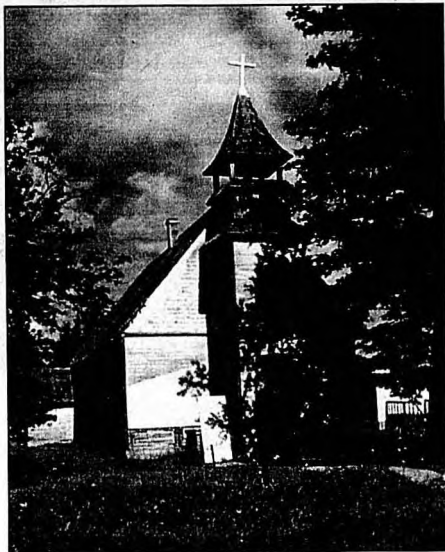
The Christ Church in Fort Alexander was the first church in the region was built more than 150 years ago, it should be restored and maintained as a heritage building.
