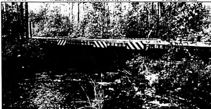
Logging road bridge over the Manigotagan River inside Nopoming Park
