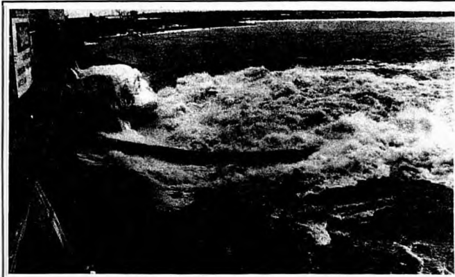
105,000 cubic feet per second passing through the Pine Falls Generating Station last Monday - more than two and a half times the normal flow. There is little danger of flooding locally.
