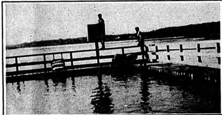
Swimming pool on the Winnipeg River
