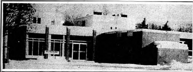
The newly completed 48 bed Pine Falls Hospital in 1963. From the Abitibi Magazine, Spring 1963. Photo Courtesy of Mathilda Smith
