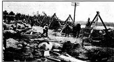
Laying of the townsite sewer, 1926
