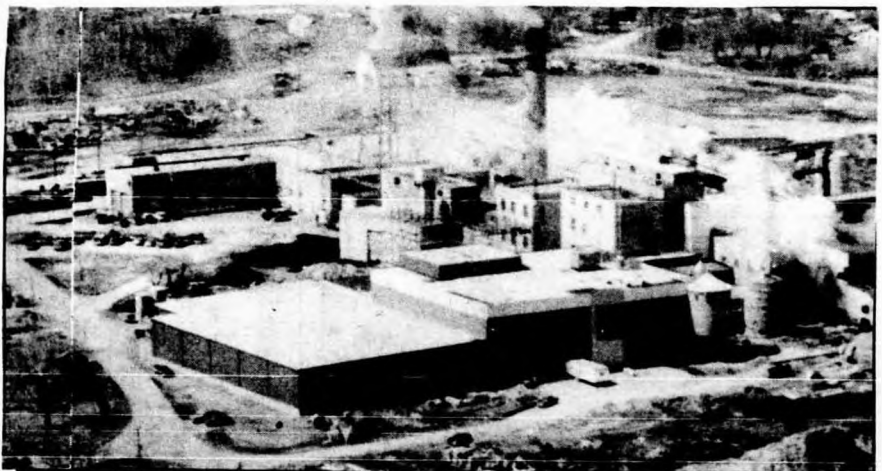
Pine Falls Paper Company Mill. The deink plant is in the foreground, the acid tank is to the back of the deink plant.
