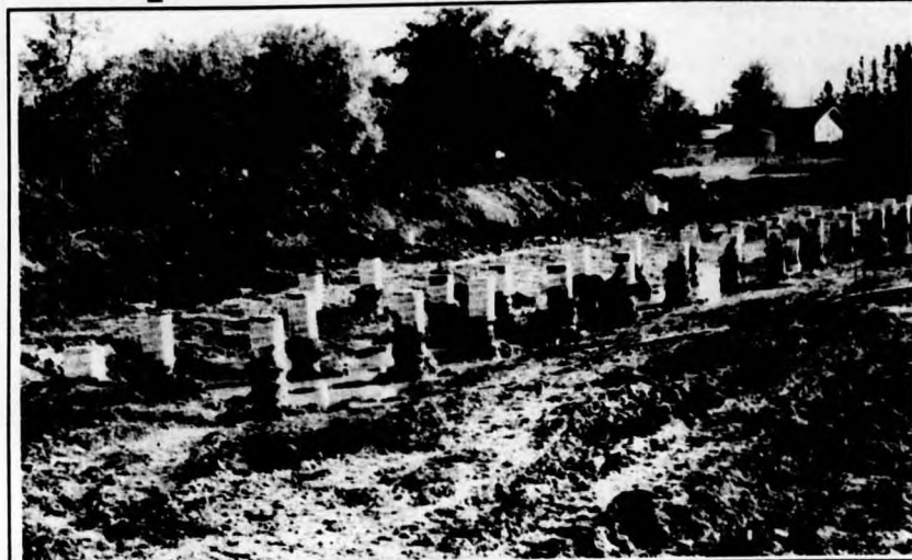
Pile foundation in place for the Powerview Seniors Complex.
