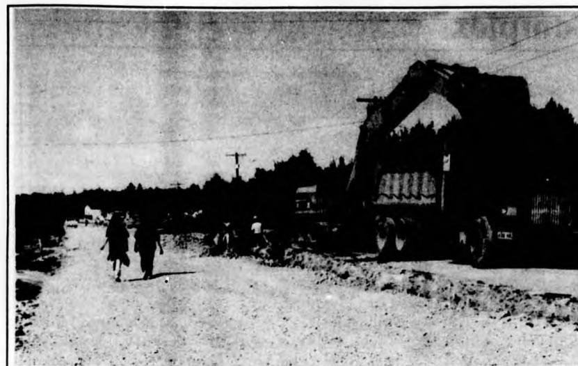
$3 Million road under construction on Sagkeeng's North Shore
