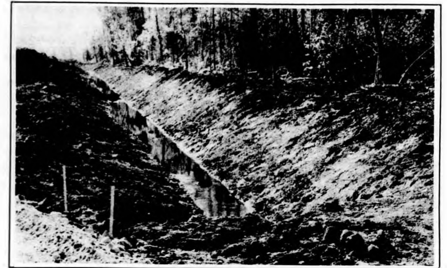
Drainage Ditch at the Effluent Treatment Site
